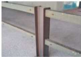
Steel beam posts + wooden rails
