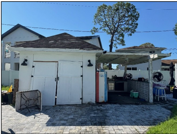
Figure 2: Historic garage with non-contributing carport.
