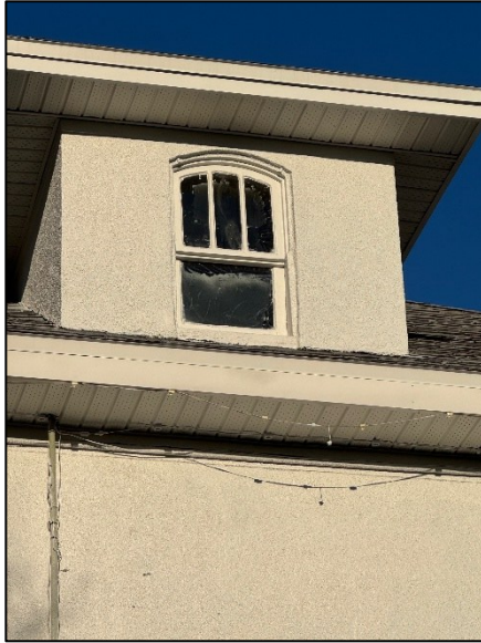
Figure 4: Original three-over-one arched windows in dormer.
