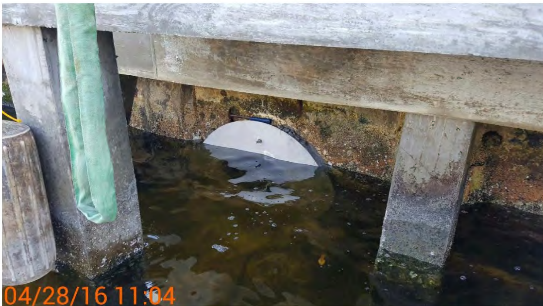
Figure 201. Completed Tideflex installation with insert
