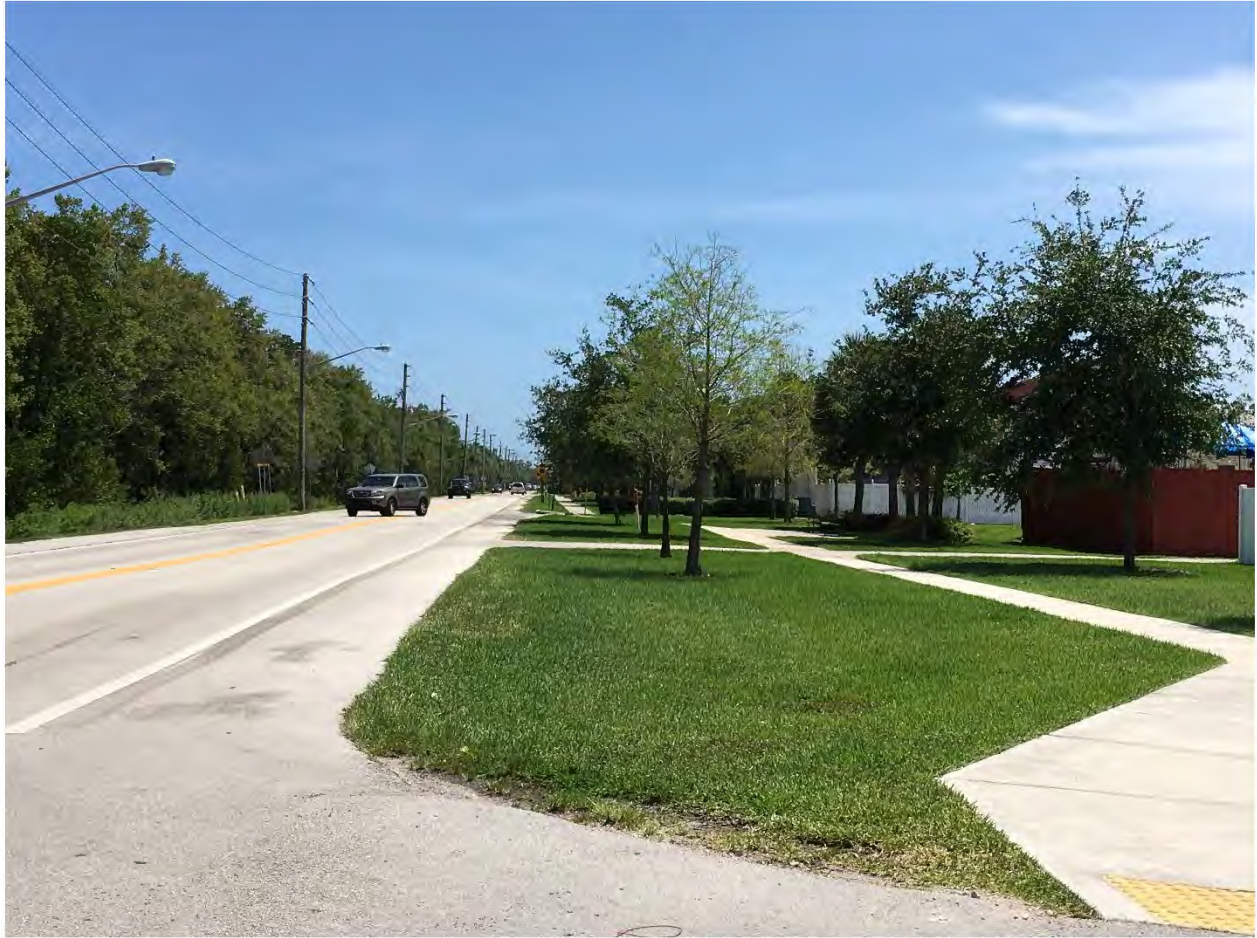
Figure 183. Roadway dry swale
