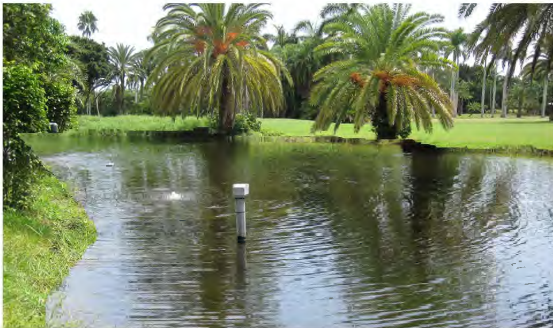
Figure 185. Aerated retention pond
