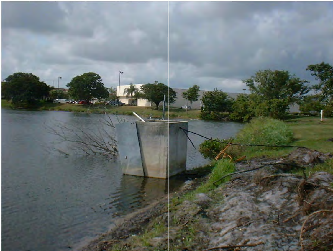
Figure 180. Detention basin with overflow
