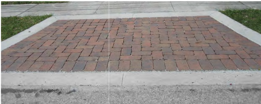
Figure 178. Example of a pervious paver driveway
