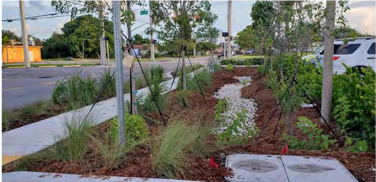
Figure 174. Photo of a bioswale pilot installation in Hallandale Beach, FL ( https://www.hallandalebeachfl.gov/ )
