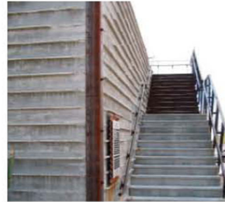
Formed concrete to look like wood siding
