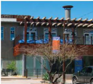
Steel, wood and wire mesh balconies
