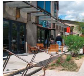
Steel + glass awnings
