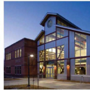
Internal building + dark sky pedestrian lighting
