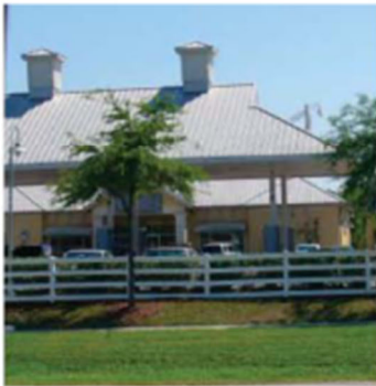
Interesting roof features
