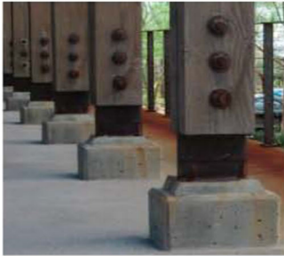
Wooden posts + steel hardware
