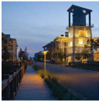
Internal building + dark sky pedestrian lighting
