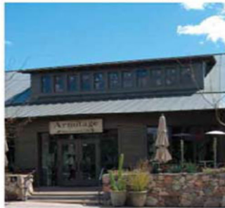
Shed-style dormer windows
