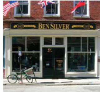
Traditional retail window fenestration
