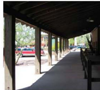
Wooden posts + corrugated metal boardwalk
