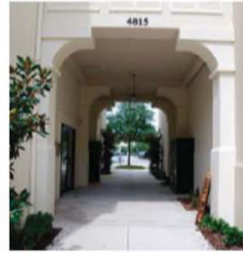
Pedestrian covered walkway
