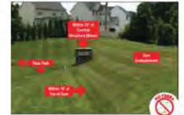
As shown in red are off-limits for trees and shrubs. They may be planted on dam embankment, which must be mowed twice a year.
