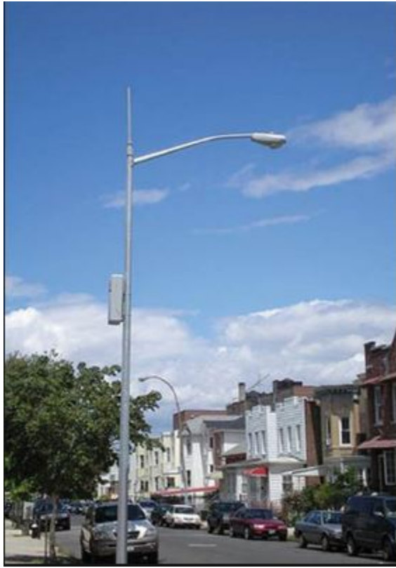
Exhibit 2. The antenna is narrower than, and in scale with the pole. This would be an acceptable design for a cobra-style light fixture.
