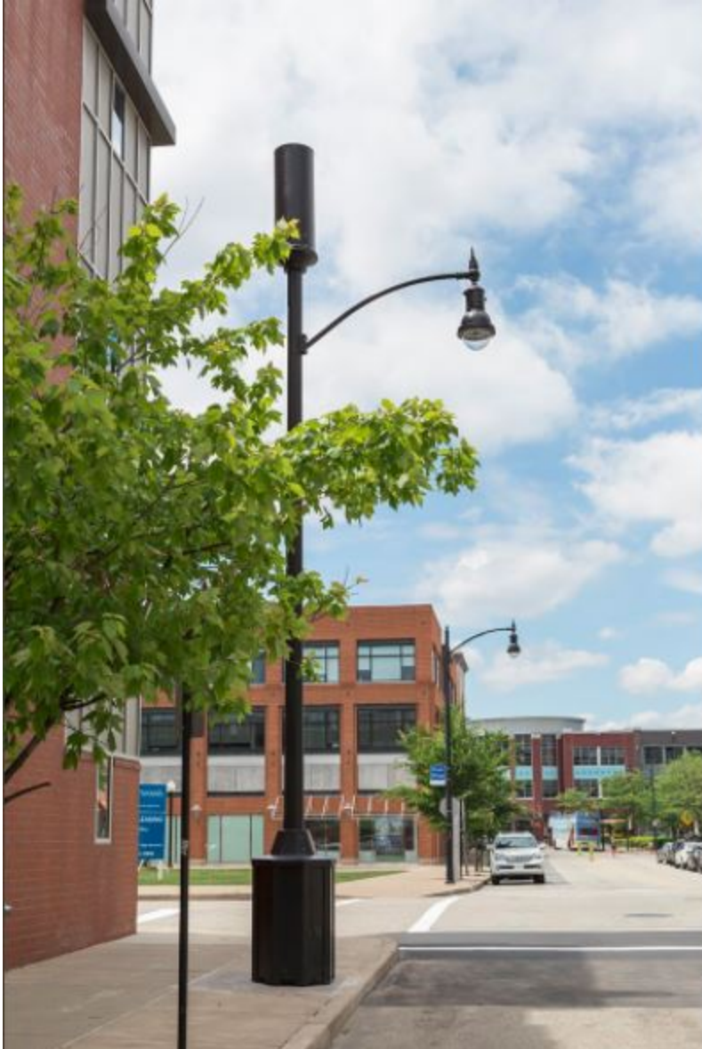
Exhibit 13. The base is out-of-scale to the size of the luminaire. In addition, the antenna is larger than the pole diameter and does not look like an original part of the pole. This design would be prohibited.
