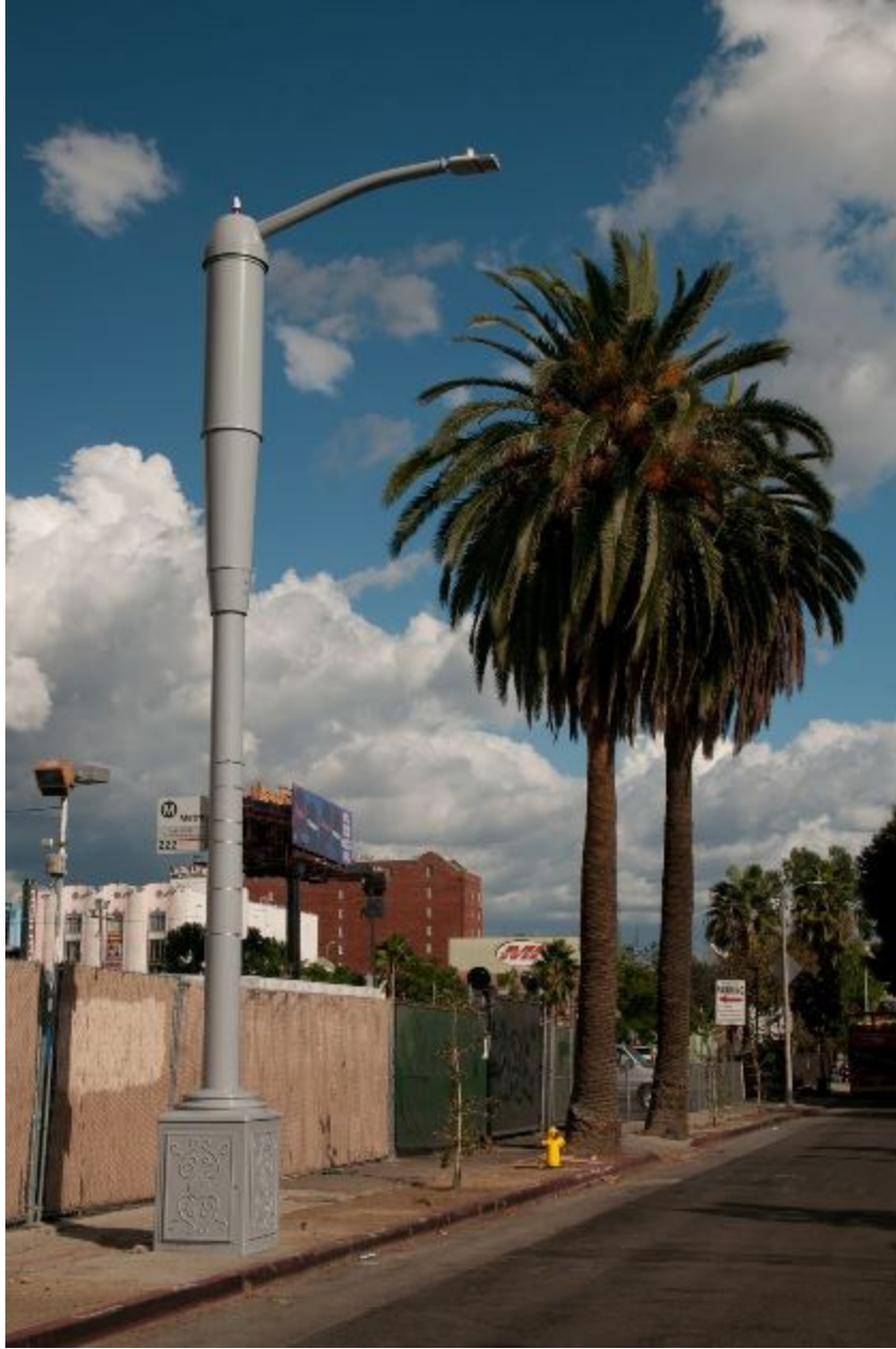
Exhibit 7. The antenna enclosure has a larger diameter than the pole, rendering it insufficiently cloaked. This design is prohibited.
