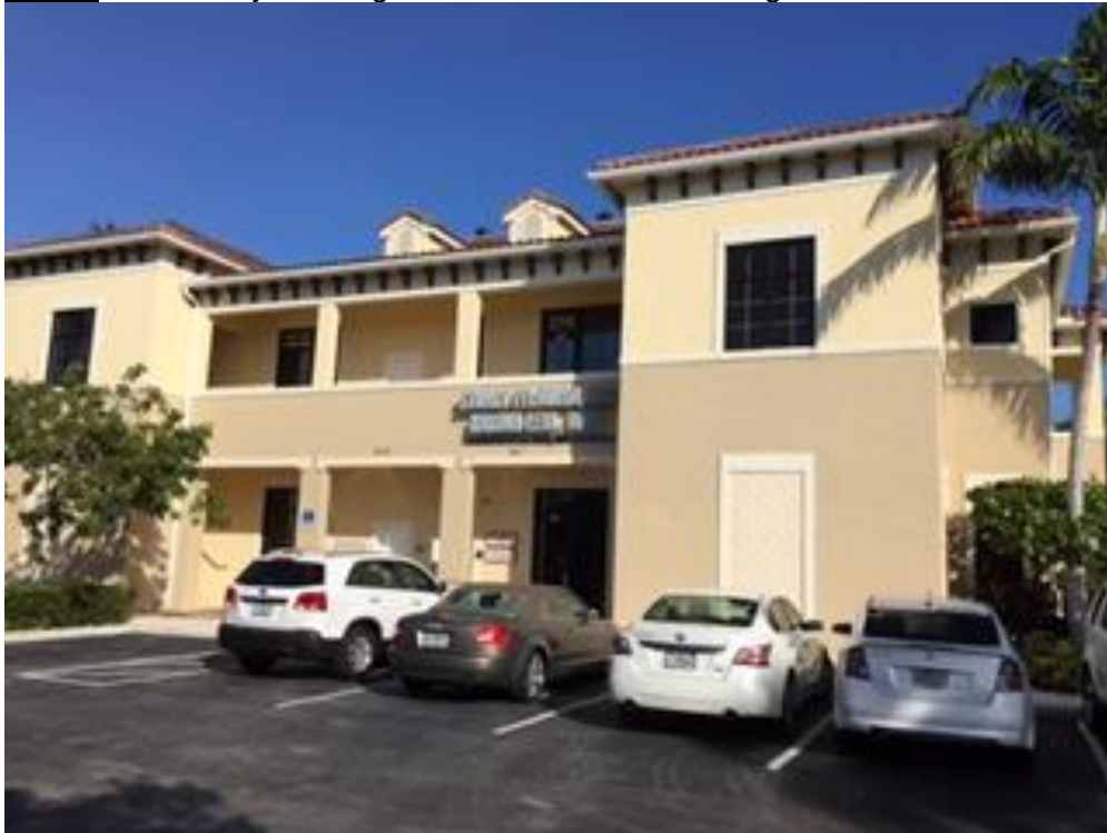
River place - 1009 W. Indiantown Road
