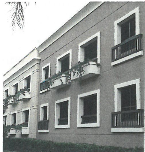
Planter boxes, window grills, protruded balconies and window framing provide the appearance of windows.
