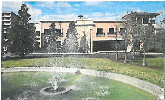
WP Towers garage with cornice, articulation, stair tower, window fenestration, planter boxes and opening framing details combine successfully.
