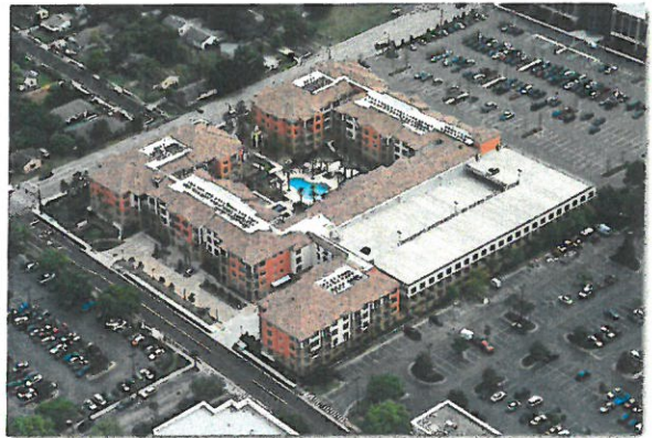
Interior location minimizes public visibility allowing landscape buffering alone to suffice.
