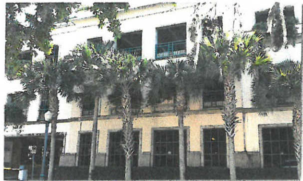
Sun Trust garage with cornice, color, window boxes, fenestration of the opening and landscape buffering combine successfully.
