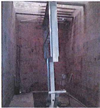
Sign's Existing Powder Coating Stripped
