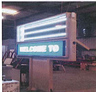
New Bulbs. Ballasts Lighting Installed
